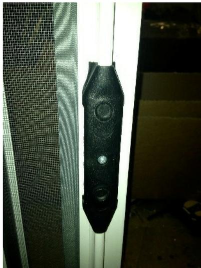
The shoot bolt is hidden behind the handle assembly and is operated by squeezing the centre handle buttons together to retract the bolt and releasing to engage the bolts into the holding catches.
