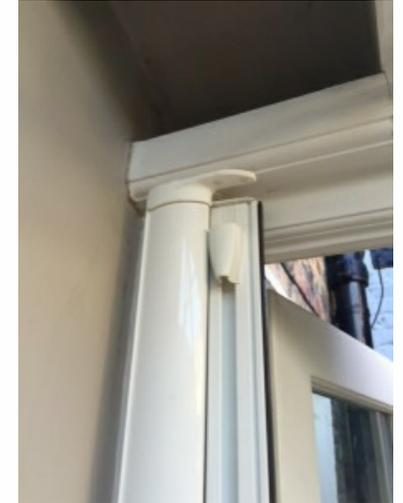
4. The top and bottom guides will now need to be installed onto the cassette and magnetic extrusion. Loosen the screws in the guide holders at the base and top of the extrusion and slide the holder up or down.
