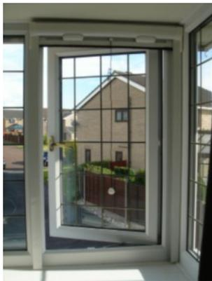
The mesh is pulled from the cassette by the bottom bar which can have handles and pull cords installed depending on your preference. At the base of this bar runs a length of brush pile which will create the seal with the window sill.
